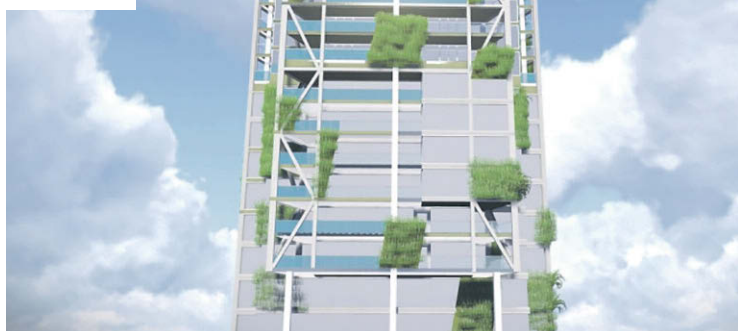
VDHG 14 East tower building
